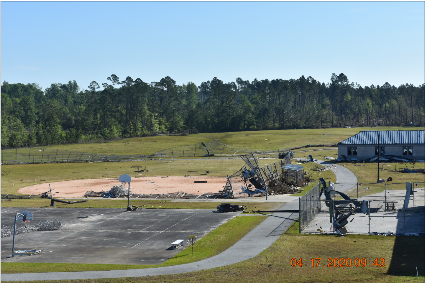
Figure 4: Tornado Damage to Perimeter Fencing and Recreation Yard at Federal Correctional Institution Estill in South Carolina, April 2020
