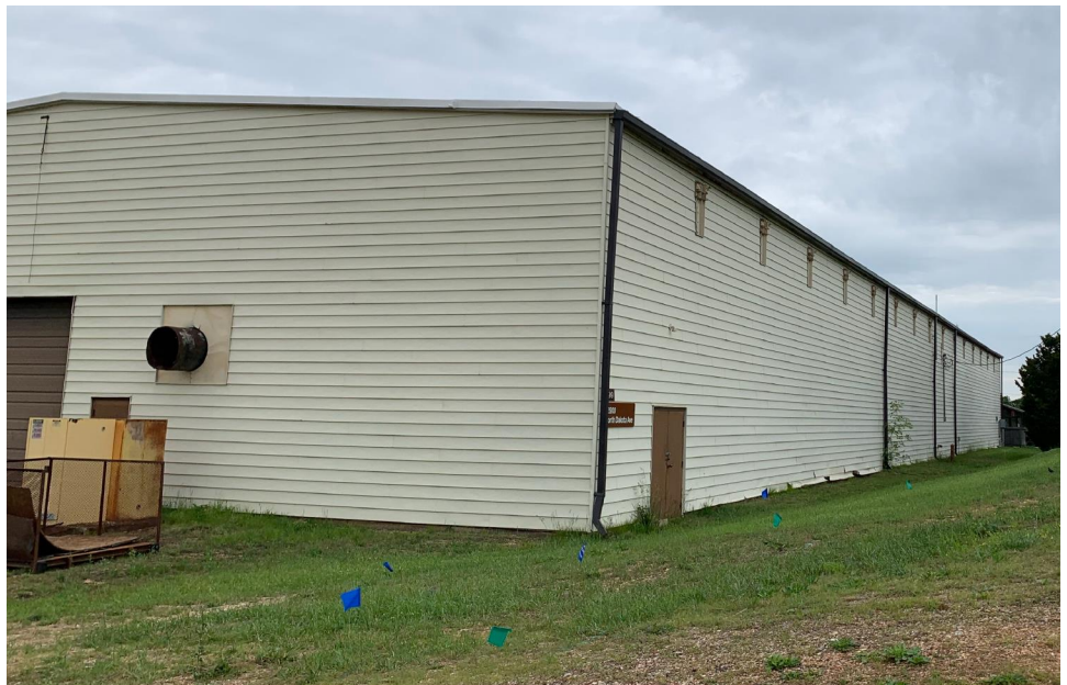
Figure 4: World War II-Era Warehouse at Fort Leonard Wood, Missouri
