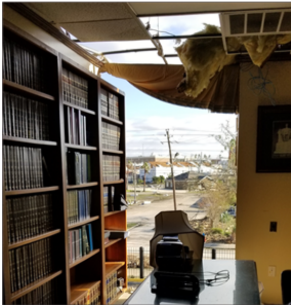
Figure 4: A Law Library at the Federal Courthouse in the Panama City, Florida, Shows Severe Damage to the Roof, Windows, and Exterior Walls After a Hurricane
