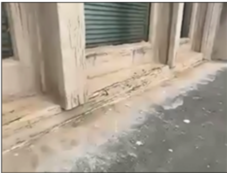
Deteriorated exterior window frame
