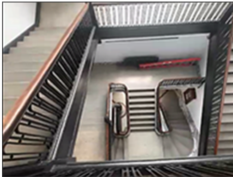
A staircase that does not meet accessibility requirements in a historic courthouse
