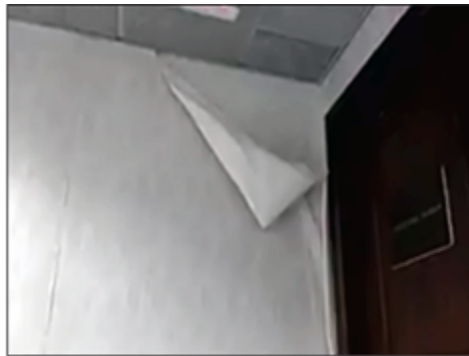
Moisture damage resulting in peeling vinyl wallpaper
