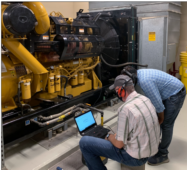
Figure 14: Headquarters-Deployed Technicians Working on a Generator at the U.S. Consulate General Dubai, United Arab Emirates
