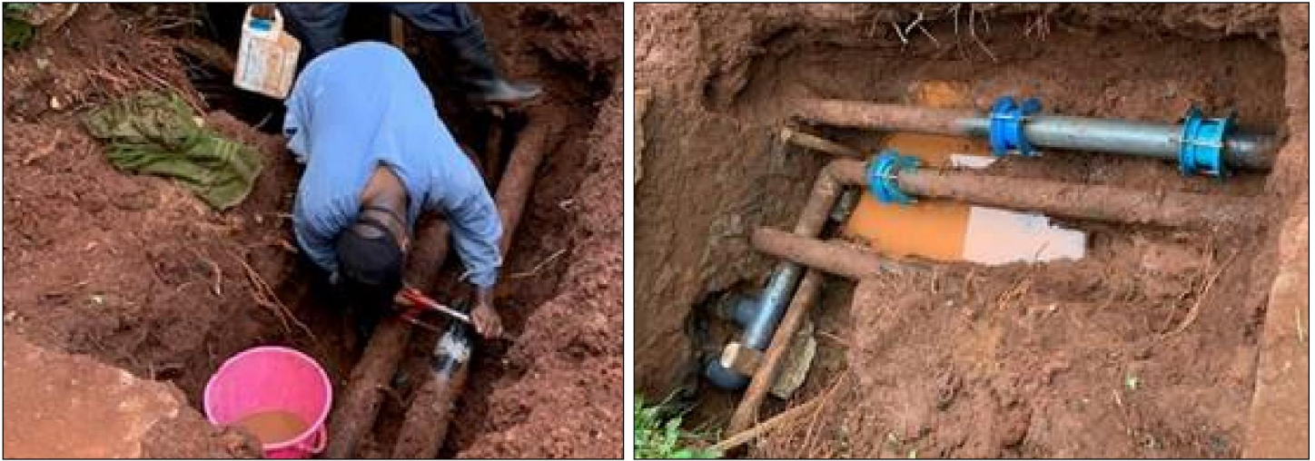
Figure 4: Pipe Repair at the U.S. Embassy in Nairobi, Kenya
