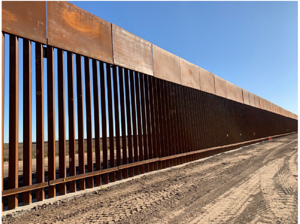
Figure 1: Border Barrier Featuring Steel Bollards in Starr County, Texas
