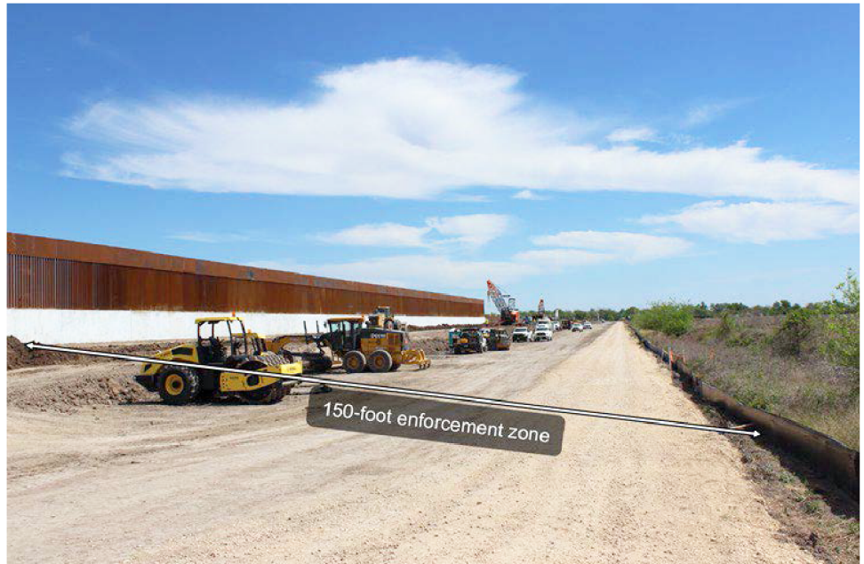
Figure 2: Border Barrier and Enforcement Zone under Construction in Rio Grande Valley Sector
