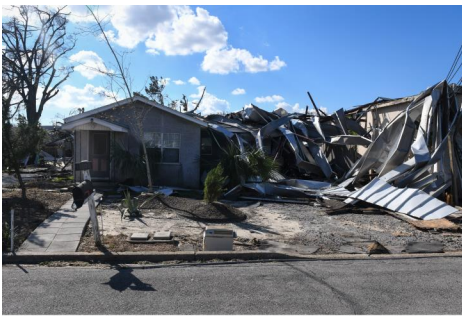
Tyndall Air Force Base, Florida (2018) Damage from Hurricane Michael
