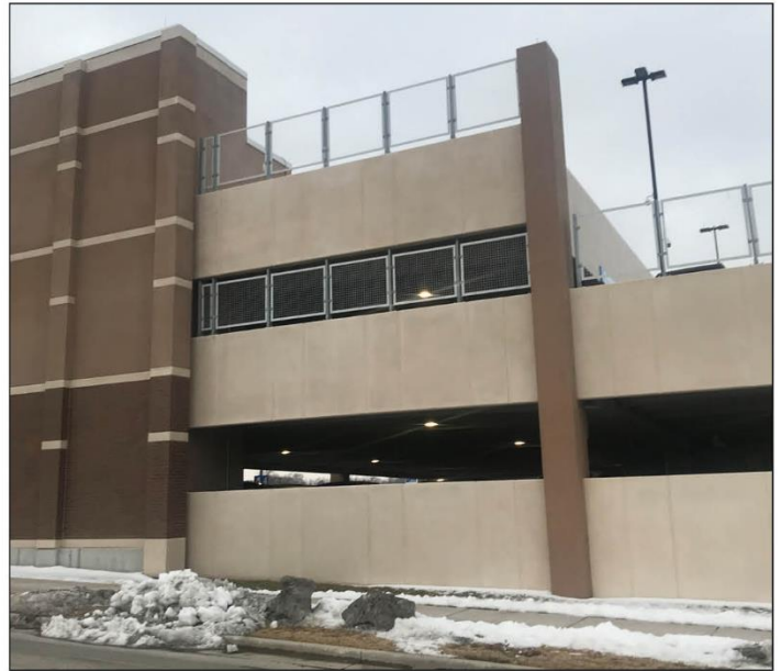
Heightened barriers at a parking garage to prevent efforts to jump off the structure.
