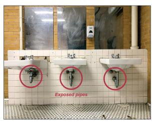
Sinks in accessible restroom have exposed pipes. Without a barrier or insulation, hot pipes could burn wheelchair users.
