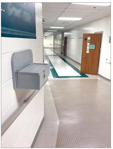
Figure 17: A Security-Related Box Protruding into a Pathway GAO Observed
