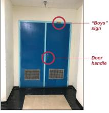
Restroom sign located too high, located on the door, and lacks raised characters or braille. Door hardware also requires pinching or grasping to open.
