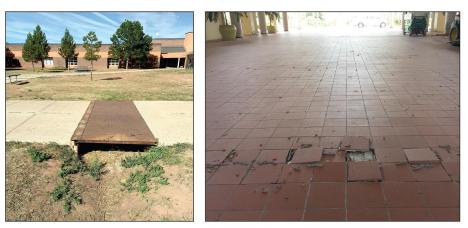
Uneven pathways (left) and large cracks in pathway surface (right).
