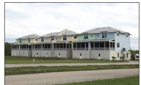
Florida homes with elevated structure and tin roofs to mitigate against wind damage.
