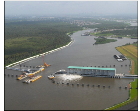
New Orleans' Hurricane and Storm Damage Risk Reduction System is comprised of numerous features including levees, floodwalls, floodgates, surge barriers and pump stations.
