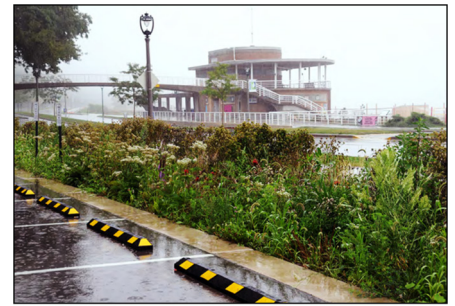
Bio-swale – a depressed catchment area planted with vegetation that captures and infiltrates runoff.
