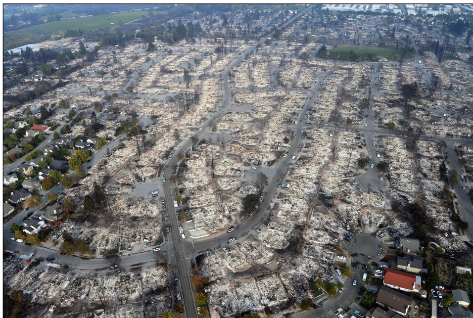
Figure 2: Aerial Photograph of Damage from Tubbs Fire, Santa Rosa, California, October 11, 2017
