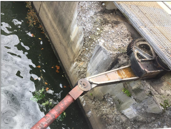
Deteriorating lock gate arm and supporting concrete at Allegheny River Lock and Dam 2 in Pittsburgh, Pennsylvania, (left) and recently rehabilitated lock gate arm at Emsworth Locks and Dams in Pittsburgh, Pennsylvania (right). Deterioration of lock gate components and surrounding concrete may lead to failure or reduced functionality of the gate and, as a result, could cause vessel delays or prevent vessels from passing through the locks.
