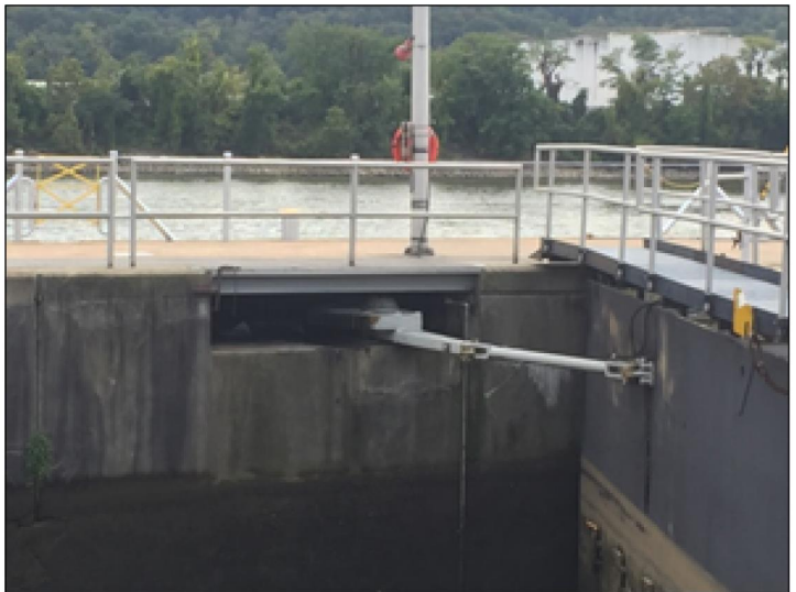
Deteriorating lock gate arm and supporting concrete at Allegheny River Lock and Dam 2 in Pittsburgh, Pennsylvania, (left) and recently rehabilitated lock gate arm at Emsworth Locks and Dams in Pittsburgh, Pennsylvania (right). Deterioration of lock gate components and surrounding concrete may lead to failure or reduced functionality of the gate and, as a result, could cause vessel delays or prevent vessels from passing through the locks.
