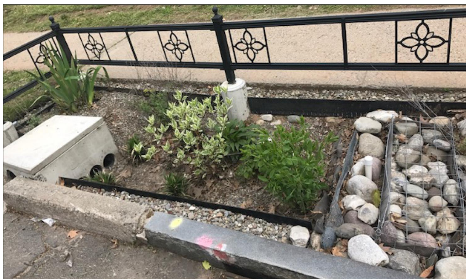
Figure 3: Bioswale in the Long Island Sound Watershed Used to Slow and Filter Pollutants from Stormwater Runoff
