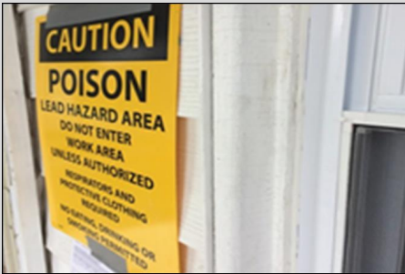
Example of a Home with Lead Paint Hazards
