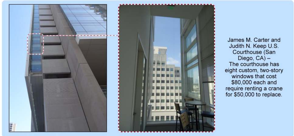
Figure 5: Large, Custom Windows in a Design Excellence Building That Increased Operations and Maintenance Costs, according to Building Managers
