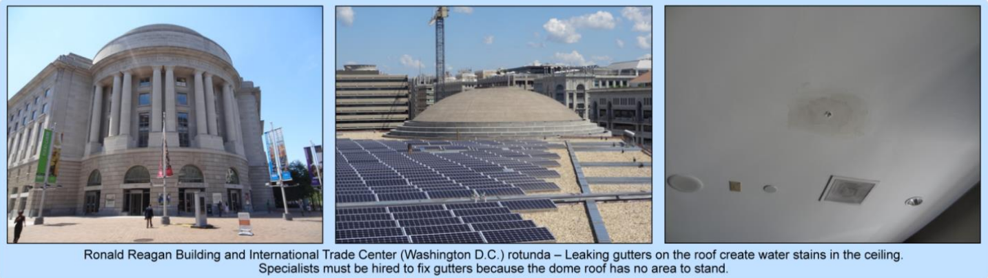
Figure 3: Separate Structure in a Design Excellence Building That Increased Operations and Maintenance Costs, according to Building Managers
