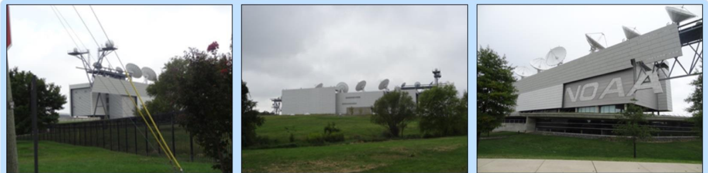
National Oceanic and Atmospheric Administration Satellite Operations Facility (Suitland, MD) – View from road (left and middle) and exterior (right).
