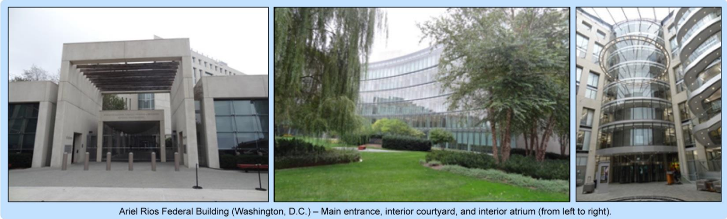
Ariel Rios Federal Building (Washington, D.C.) – Main entrance, interior courtyard, and interior atrium (from left to right).
