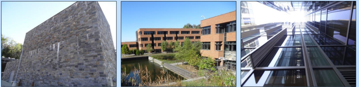
Douglas A. Munro Coast Guard Headquarters Building (Washington D.C.) – The building façades incorporate multiple materials, including two types of stone (left), brick (right), and glass and steel (bottom), which are difficult to clean. Some sections require additional equipment, leading to expensive cleaning costs.
