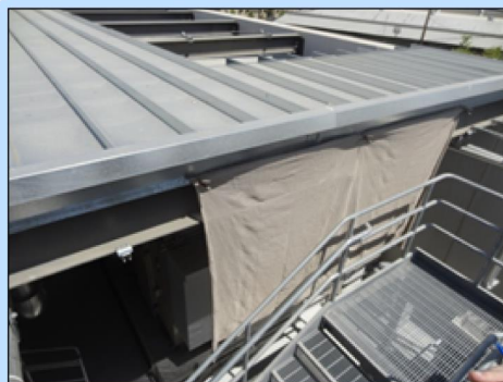
Bakersfield Federal Courthouse (Bakersfield, CA) – The mechanical systems are placed on the roof and exposed to extreme environmental conditions. Building managers have hung makeshift drapes in an attempt to protect these systems from overheating (left). Sand can clog the air intake fans for the building’s air conditioning unit (right).
