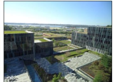
Douglas A. Munro Coast Guard Headquarters Building (Washington, D.C.)
