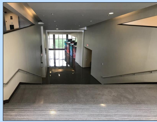
Las Cruces U.S. Courthouse (Las Cruces, NM) – Special lift required to replace lights in the grand stairway. To minimize costs, lights are replaced once a year.
