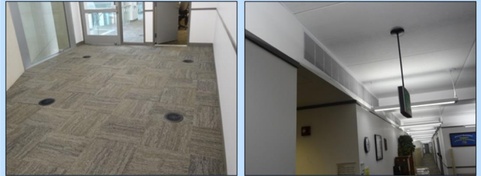
Ariel Rios Federal Building (Washington, D.C.) – The position of the building's heating, ventilation, and air-conditioning system leads to increased maintenance, repair, and energy costs. The air-supply in the raised floor (left). The air-return in the ceiling (right).
