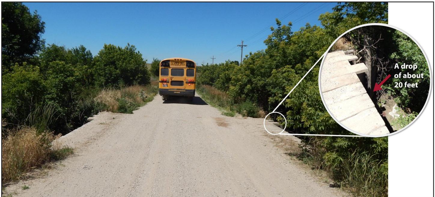
Figure 9: School Bus Route Traversing a Wooden Bridge on the Pine Ridge Reservation
