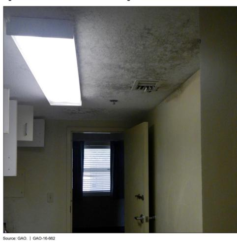
Figure 6: Barracks Vacated Due to Mold at Eglin Air Force Base
