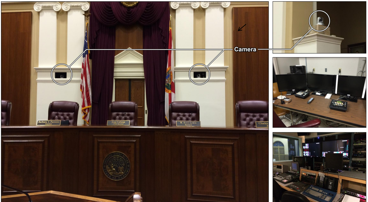
Figure 7: Cameras in the Supreme Court of Florida's Courtroom, the Court's Video and Audio Control Room, and WFSU-TV's Production Room
