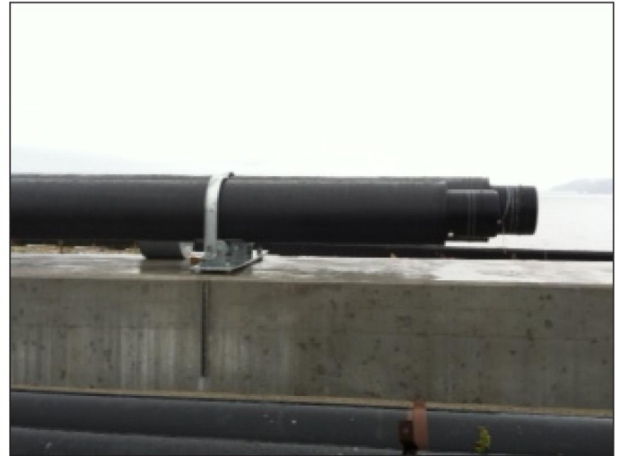
New, strengthened water lines being installed
