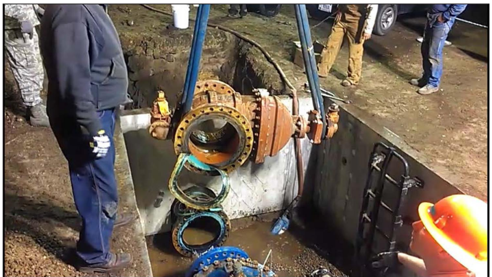
Figure 6: Repairs to a Potable-Water Pipe on Vandenberg Air Force Base
