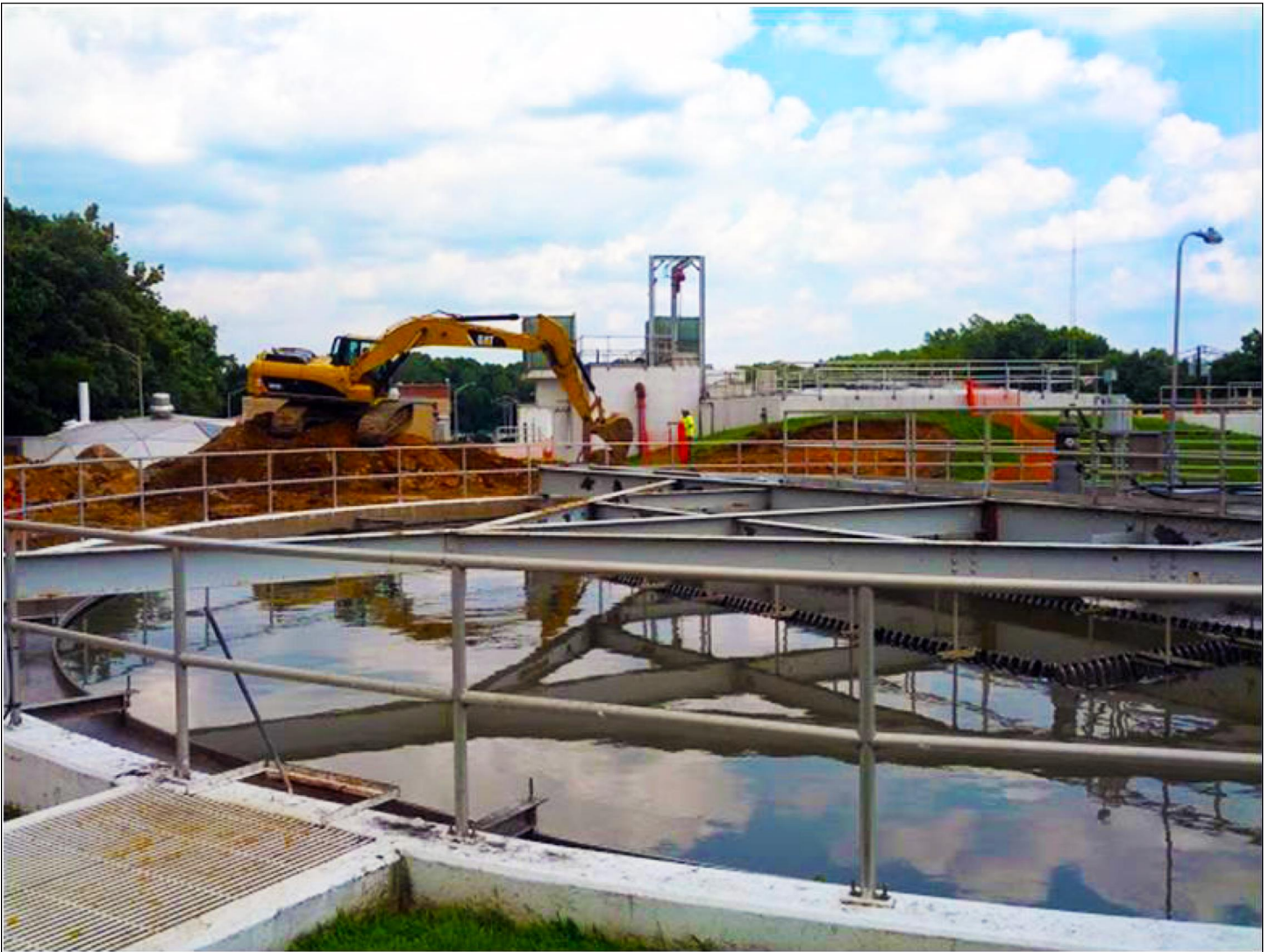
Figure 1: Upgrades to a Wastewater Treatment Plant in New Jersey
