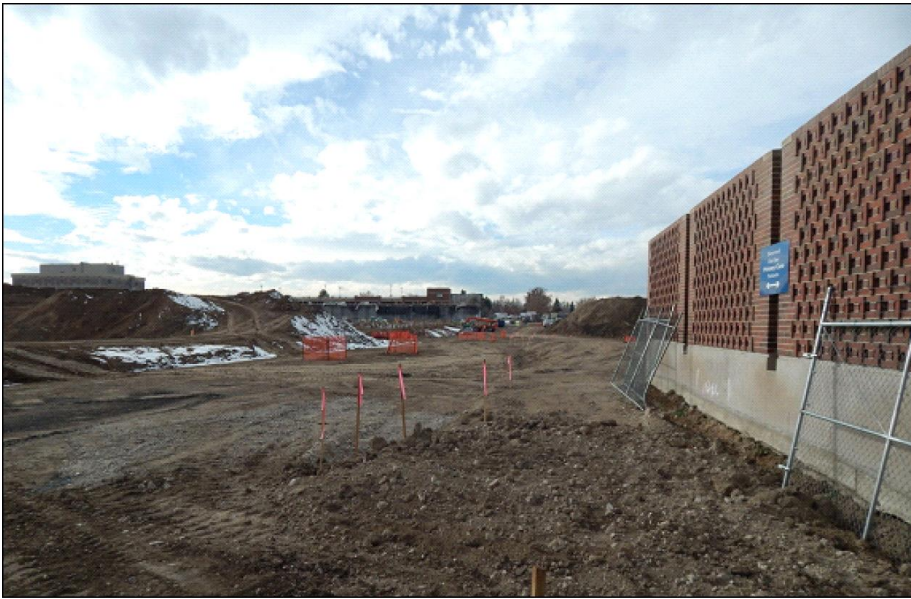
Figure 5: Demolished Site Listed as Provider's Practice Location
