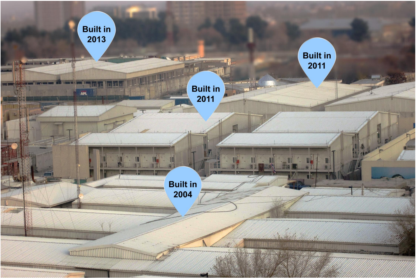
Figure 7: U.S. Embassy Kabul, Temporary Facilities
