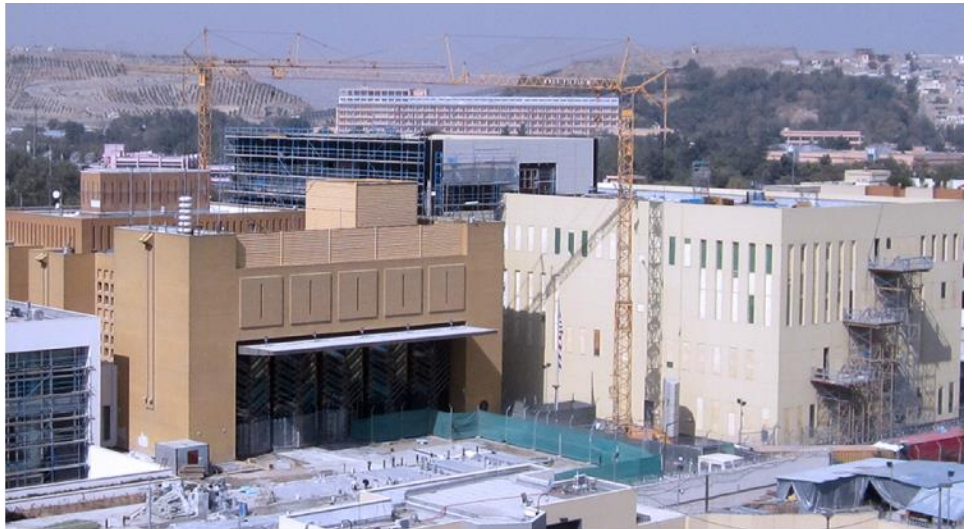
Figure 5: U.S. Embassy Kabul, West Compound, 2006 Chancery and Office Annex B
