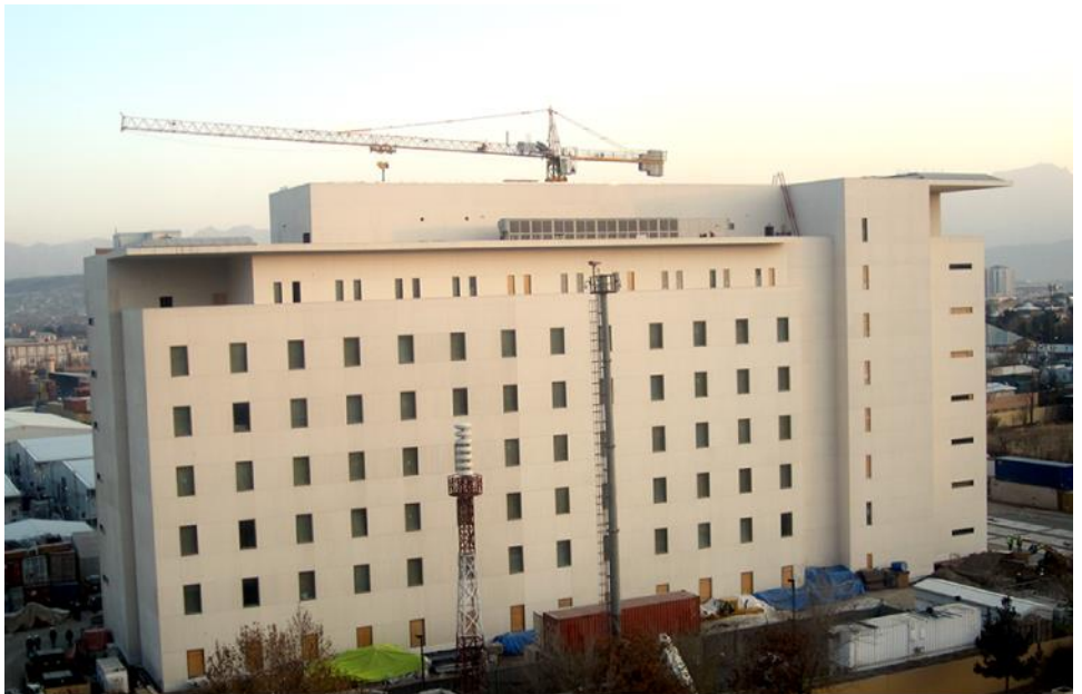
Figure 6: U.S. Embassy Kabul, East Compound, Apartment Building 1
